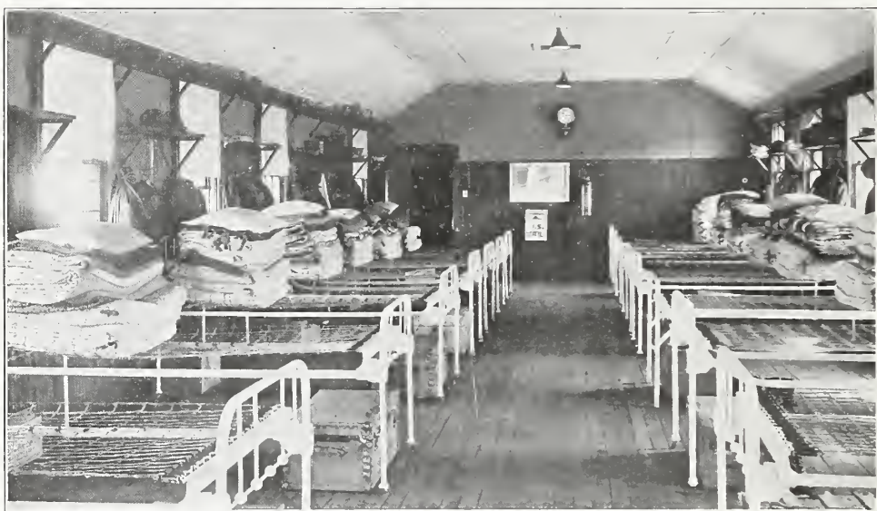
FIG. 128.—Enlisted men's barracks, Post Hospital, Barron Field, Texas.
